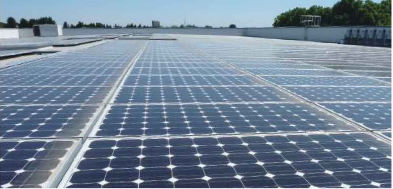
Centre commercial (ERP) - France
