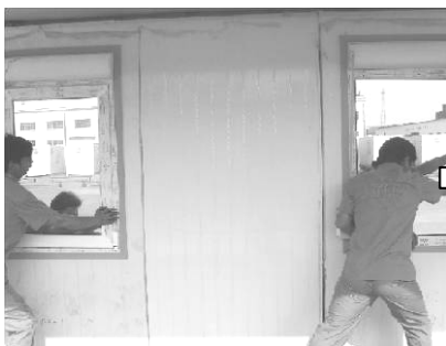
Insert the end small panel
