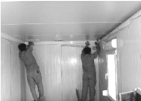
Install the top and corner PVC lining
