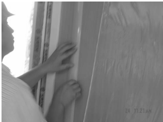
Install cover lining
