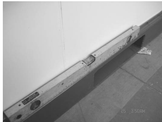
Adjust the bottom side rail
