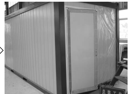
the Installed house end side
