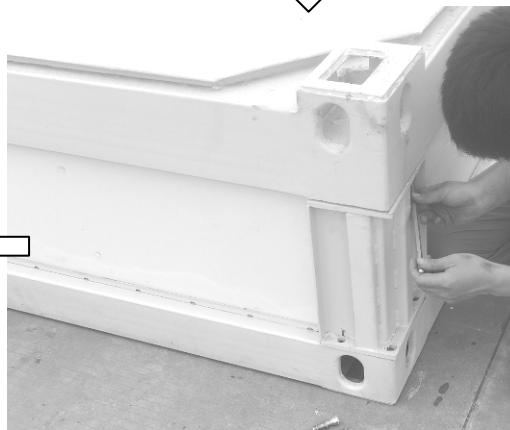
Dismantle the bolts from the short posts
