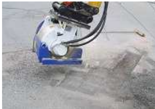
EX Standard Patch Planer mounted on Skid Steer Loader
