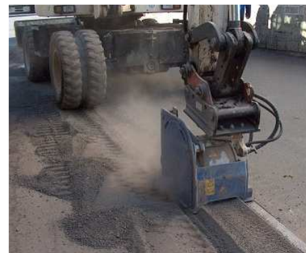
EX Standard Patch Planer mounted on Skid Steer Loader
