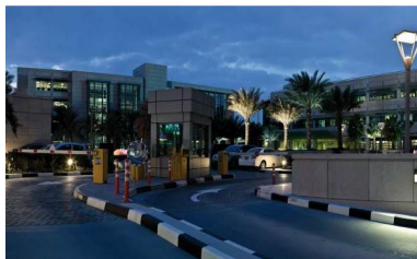
American Hospital VAE - Dubai
