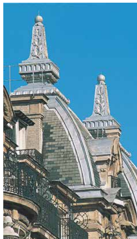
Avenue Montaigne, Paris (75)
