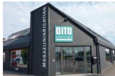
BITO Systems in Belgium
