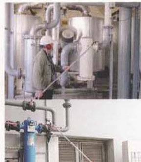
Picture above Leak detection by an air sound detector
