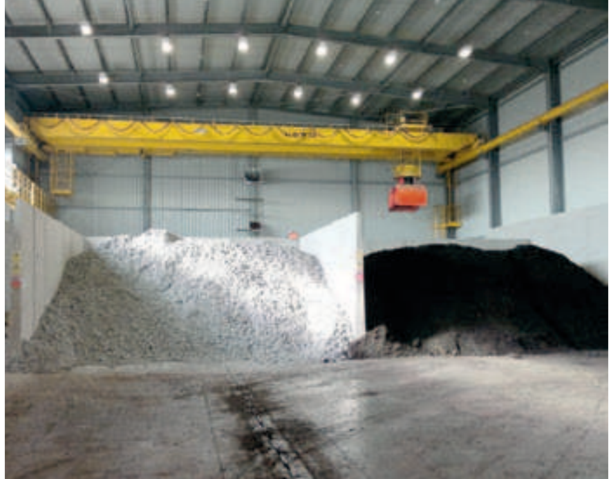
BEUMER system technology for the warehouse
