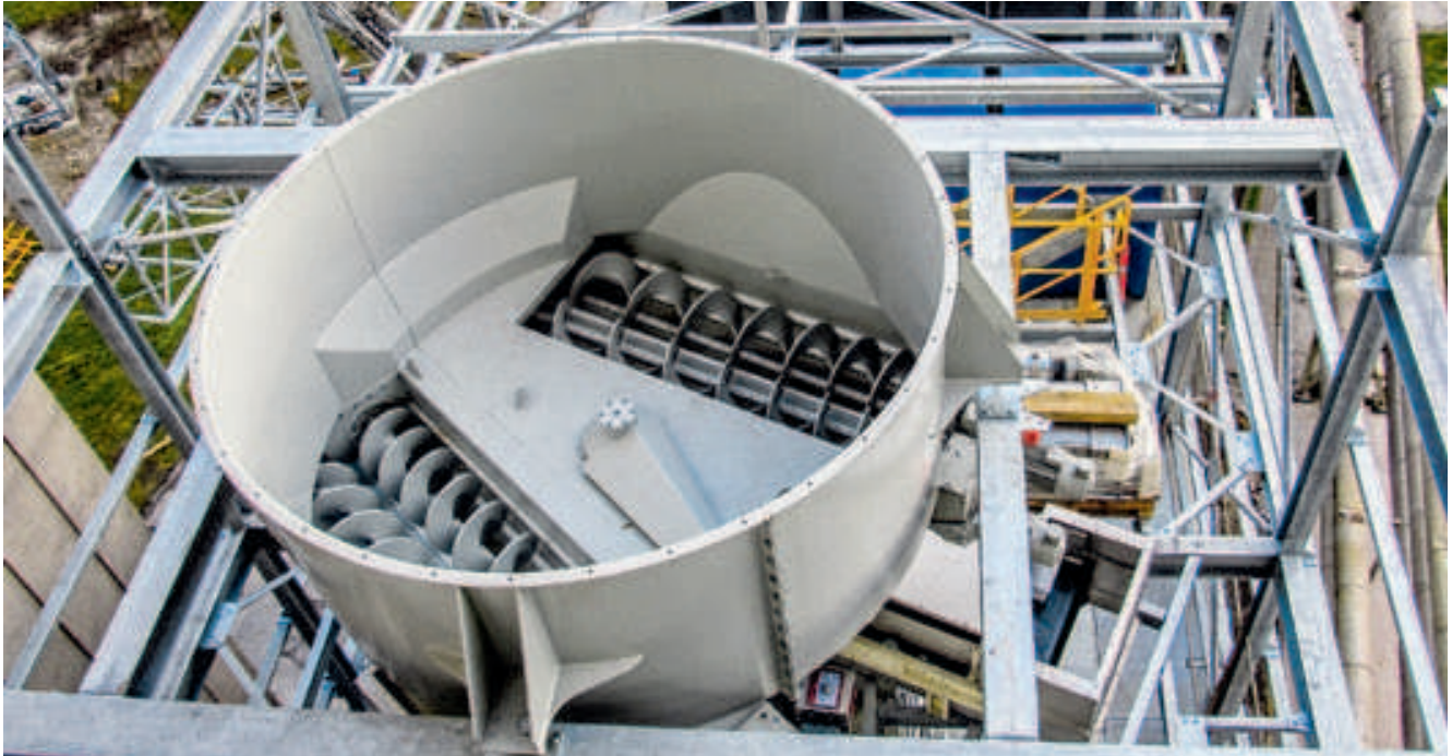
Intermediate bin with agitator and helix prefeeders
