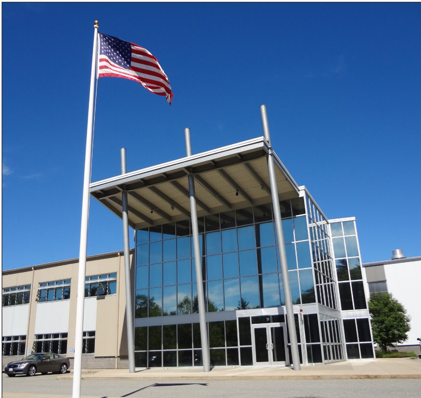
Weir Valves & Controls USA in Ipswich, MA
