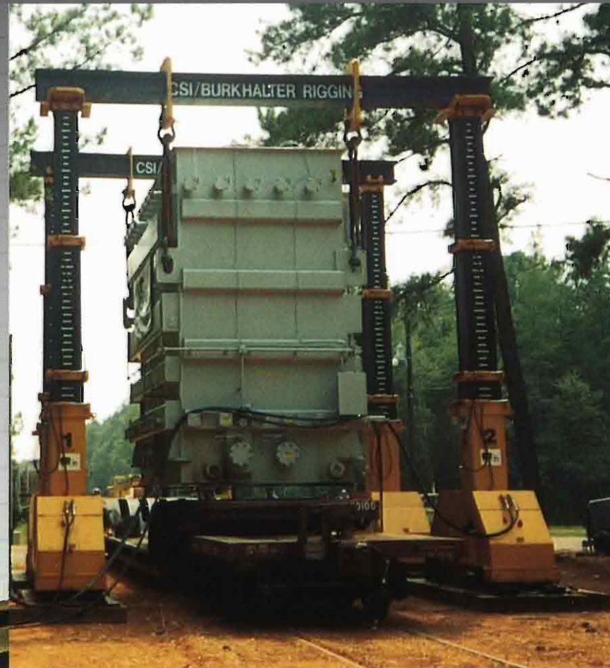
Rail siding transformer lift
