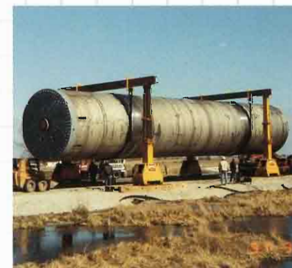
Module units handling a long load
