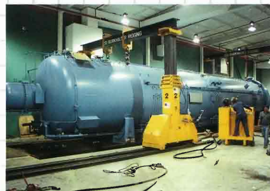
Installing a long load in a confined area
