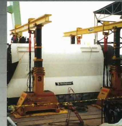
590 ton generator lifted and suspended 14 days for maintenance
