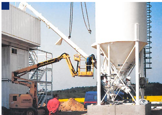
Installation of the cement silos and screw conveyors
