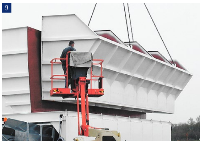
Assembly of the aggregate batcher (consisting of three transport units)
