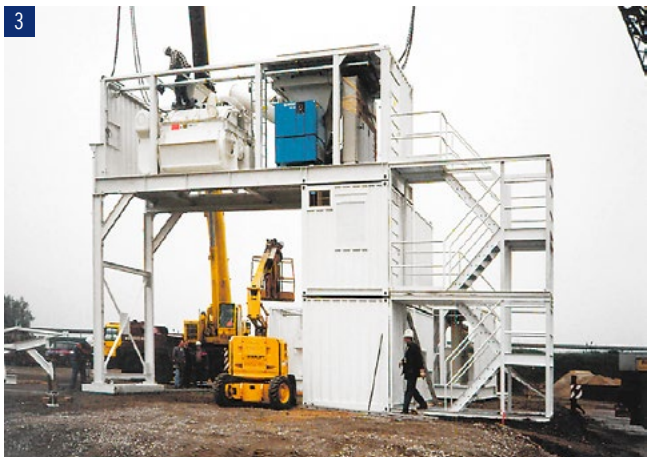
3 Positioning the mixer module on the container base. Fastening with twist-lock elements
