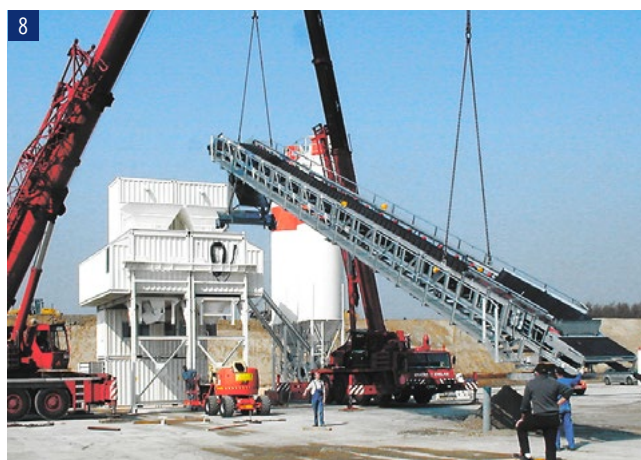
Positioning the inclined belt conveyor
