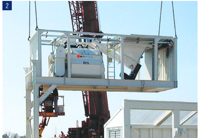
2 Installation of the support beam on the mixer module
