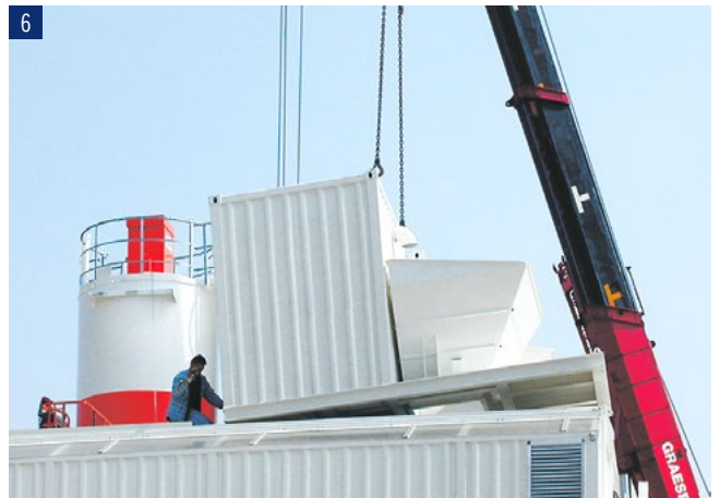
6 Installation of the weighing module
