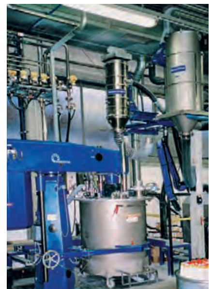
Vacuum conveyor for conveying pigments in the manufacturing of paint.
